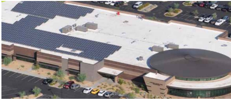
Figure 13. Grid-Connected Commercial System
