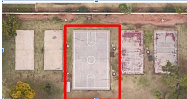
Figure 29. Location of the Basketball Court
