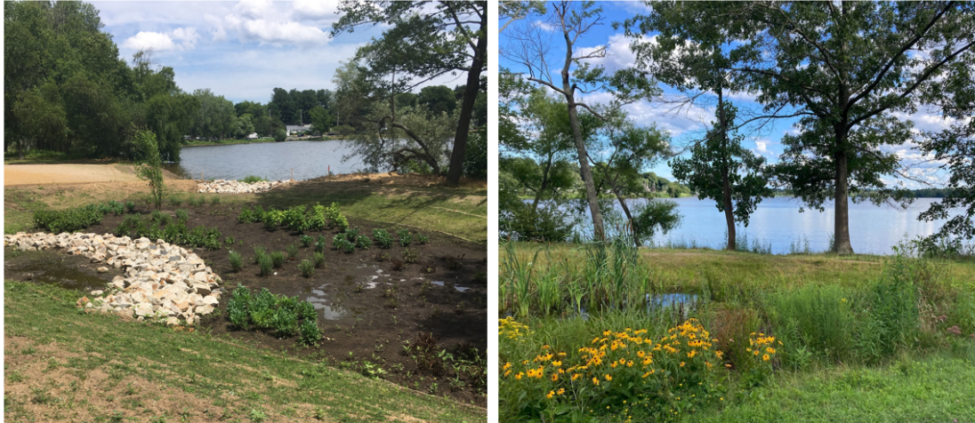
Figure 7: Example of bioswale in Wakefield, Massachusetts. Initial construction (left) and vegetation growth after one year (right).
