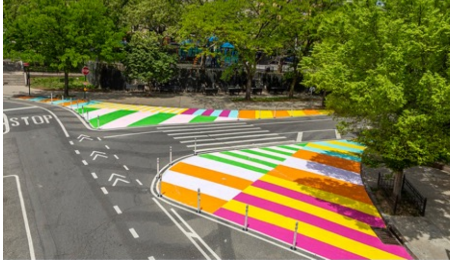
Figure 4: “Daylighting” with Curb Extensions in Hoboken
