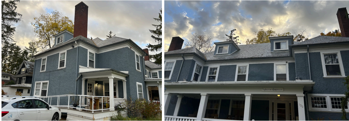
Figure 1: Exterior of Triphammer Cooperative (Source: Maya Yu)
